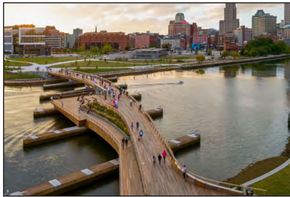
PROVIDENCE RIVER PEDESTRIAN BRIDGE INFORM STUDIO
